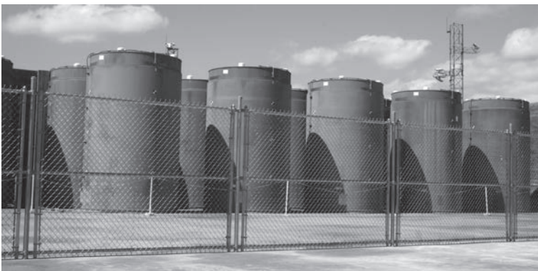
Figure 3: dry cask storage of spent nuclear fuel at the Vermont Yankee site in the USA (photo: Entergy)
